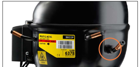
Fig.3 NLE compressor with copper connectors
